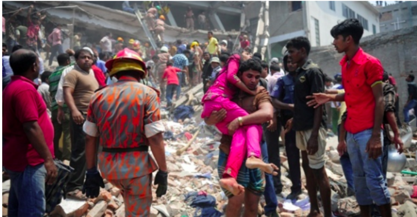
A Bangladeshi volunteer carries an injured garment worker from the Rana factory near Dhaka, Bangladesh, after the 8-story building collapsed Wednesday. (Munir Uz Zaman/Getty)
